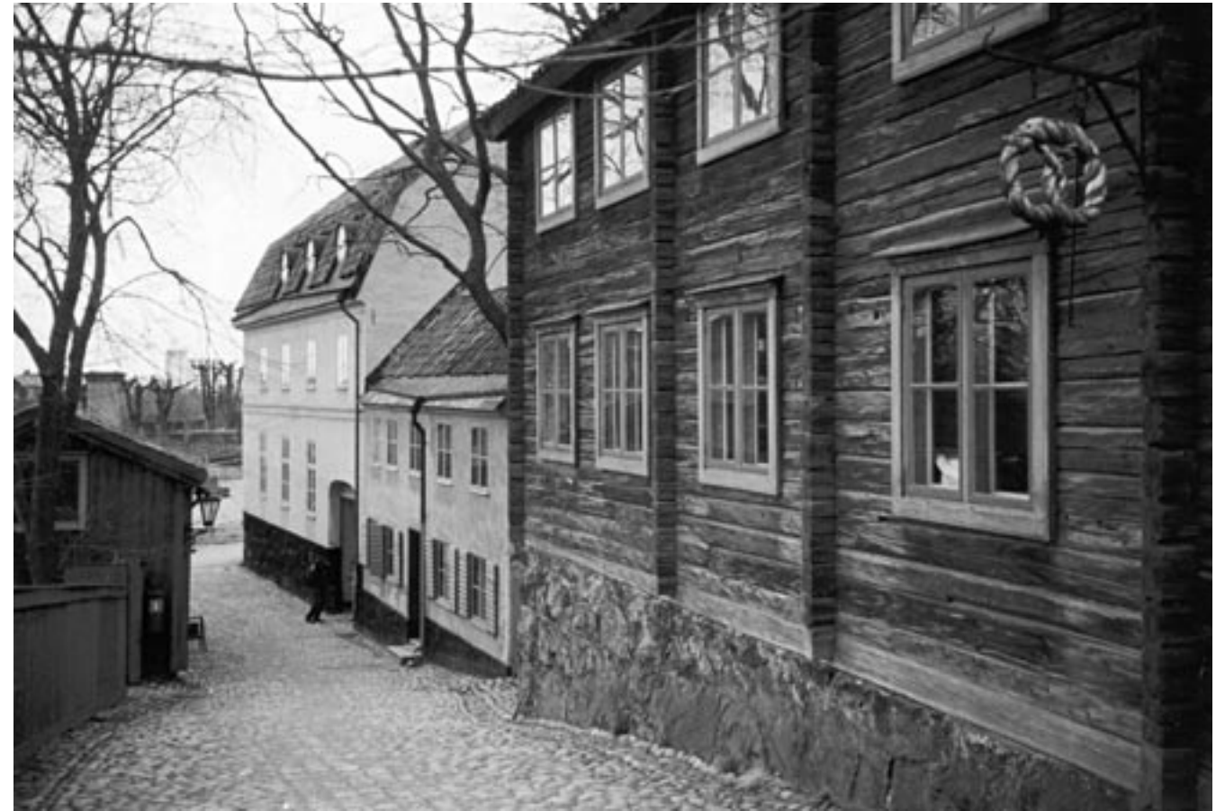
Wooden house on stone foundation in a skansen, Stockholm, Sweden
